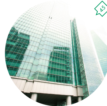
The wall of IZUMI GARDEN
